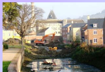
Working on the canal by the Council Offices at Ebley Mill
